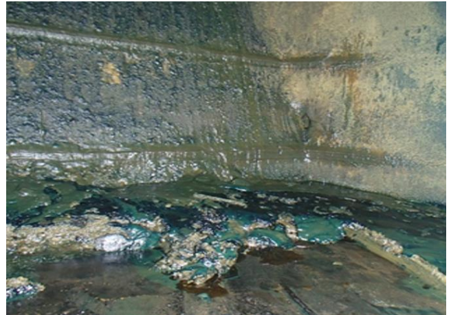
Example of solid wax deposits on tank bottoms
