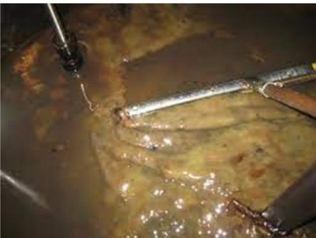
Sludge created by bio-fuel build-up being scraped from the bottom of a tank.
